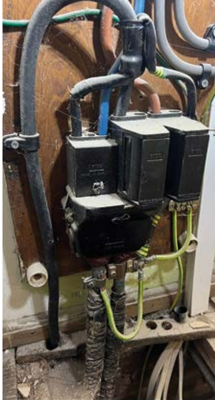
↑ Figure 4 – Intake position with two cut-out fuses
