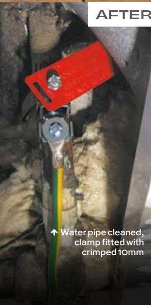
↑ Water pipe cleaned, clamp fitted with crimped 10mm
