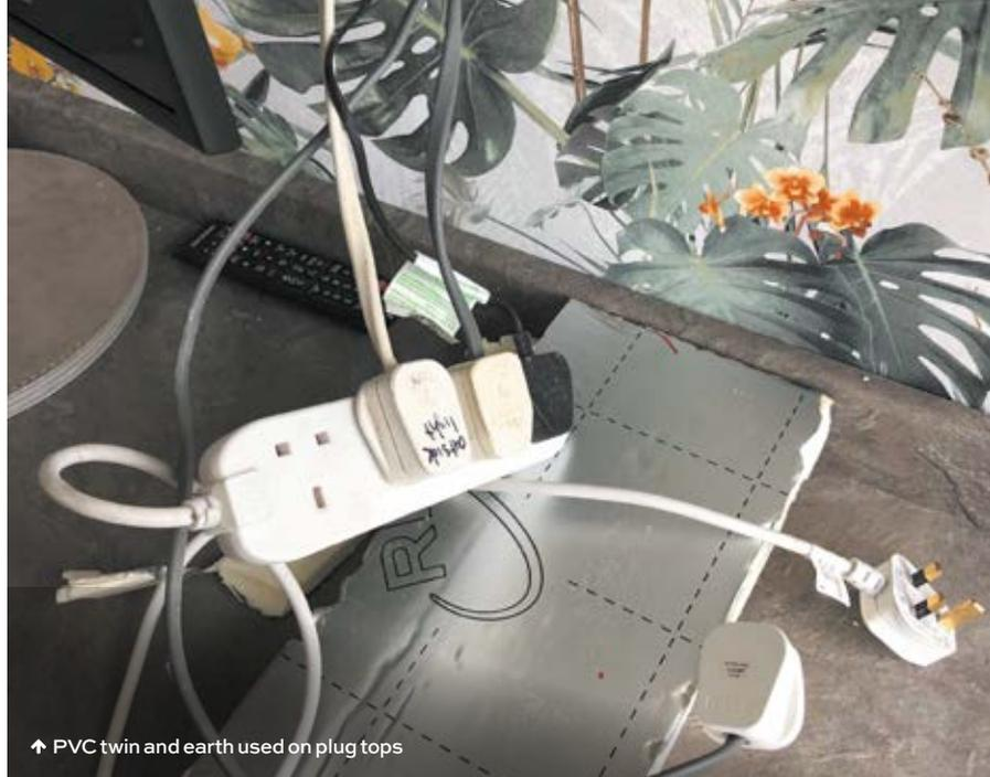
↑ PVC twin and earth used on plug tops
