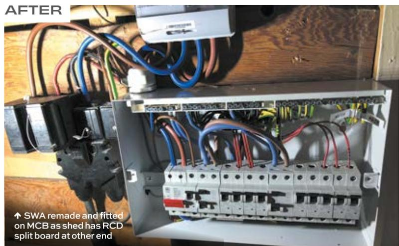
↑ SWA remade and fitted on MCB as shed has RCD split board at other end
