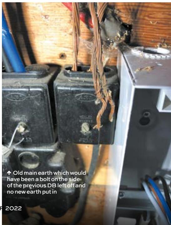
↑ Old main earth which would have been a bolt on the side of the previous DB left off and no new earth put in
