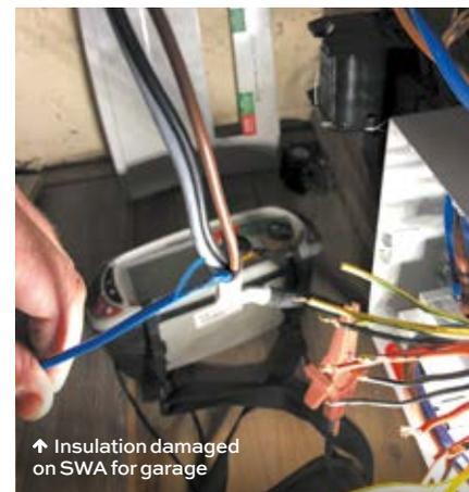
↑ Insulation damaged on SWA for garage
