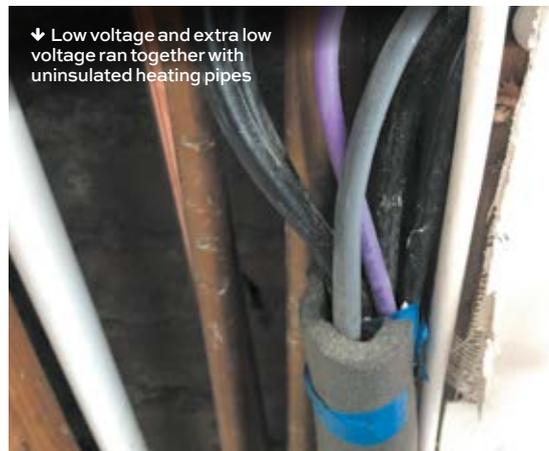
↓ Low voltage and extra low voltage ran together with uninsulated heating pipes
