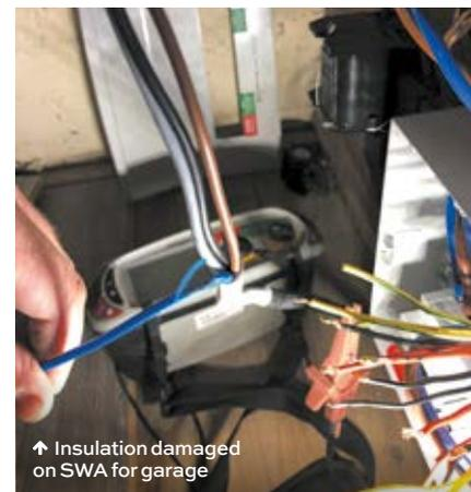
↑ Insulation damaged on SWA for garage
